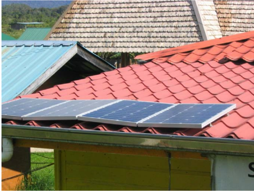
Figure 2-2-4: Solar panel installation on barrio telecentre's rooftop
