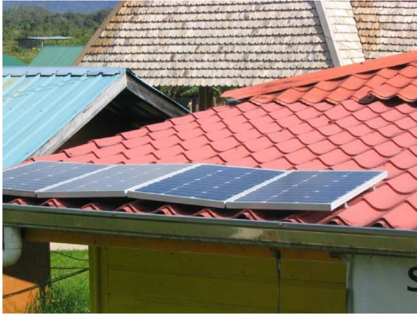
Figure 2-2-4: Solar panel installation on barrio telecentre's rooftop
